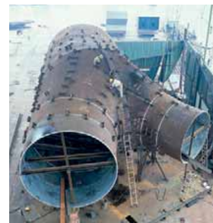
Penstock branching section
